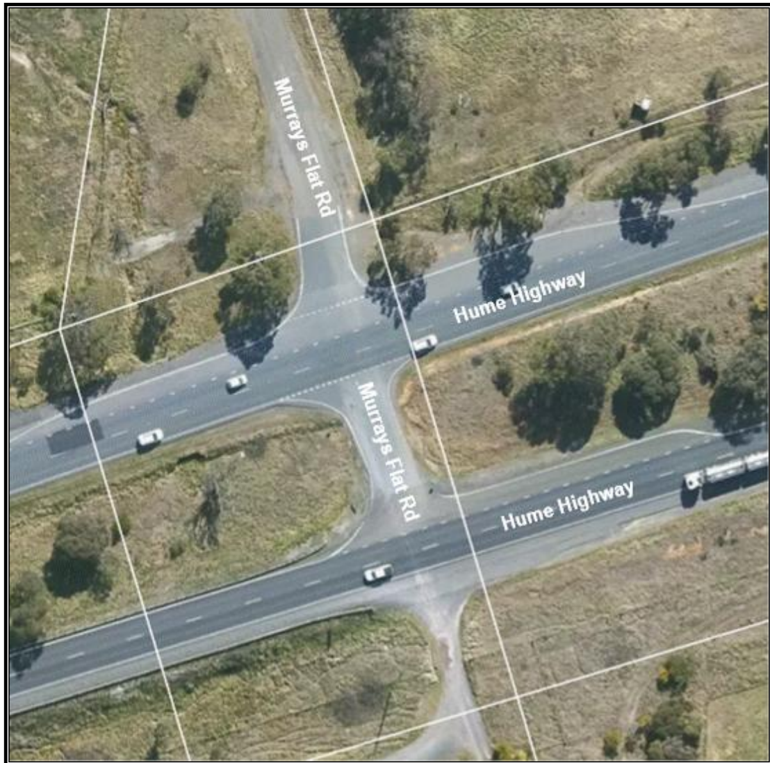
Photo 3: Aerial photo of the 2-staged intersection with Hume Highway and Murrays Flat Road
